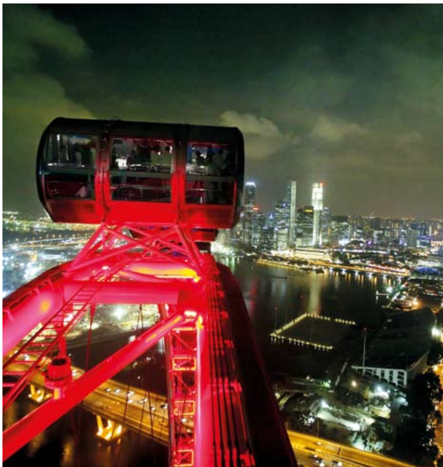
The Singapore Flyer is also the first installation in the world to be controlled by a Wireless DMX infrastructure, which can offer possible lighting scenes for the Flyer to suit themes and occasions.
