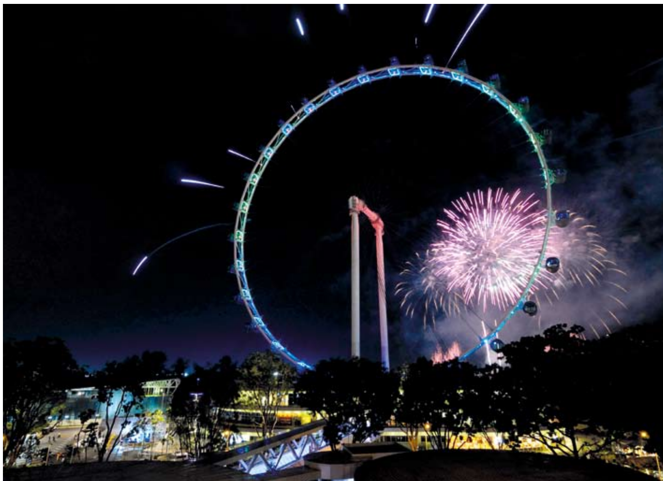
As it involves thousands of DMX channels, it is essential to make sure that all the LED fixtures receives 100 percent signal when the wheel is on the move.
